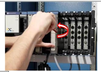
While holding the BLK connector to keep it straight, 2 unscrew the fast action screw to unsecure the BLK connector.
