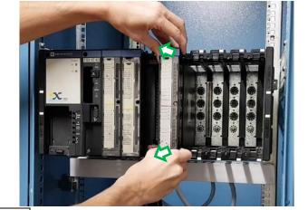
Once the central screw is completely unscrewed, remove the BLK terminal block by pulling it straight (do not tilt the terminal block out)
