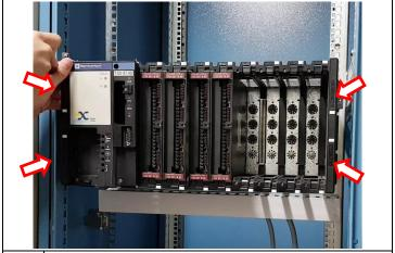
When all BLK connectors are removed from the rack, unsecure the rack using the screws and remove it.
