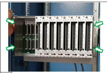
Install the FIRELEC BC-11406 in place of the legacy TSX file and secure it with the screws.
