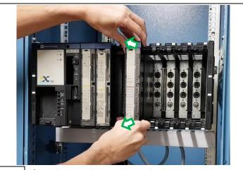
Once the central screw is completely unscrewed, remove the BLK terminal block by pulling it straight (do not tilt the terminal block out)
