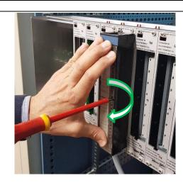
While holding the BLK connector to keep it straight, screw the fast action screw to secure the BLK connector.
