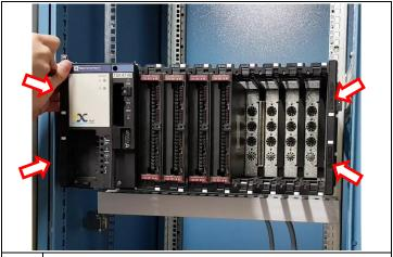
When all BLK connectors are removed from the rack, unsecure the rack using the screws and remove it.
