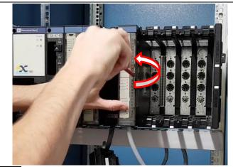
While holding the BLK connector to keep it straight, unscrew the fast action screw to unsecure the BLK connector.
